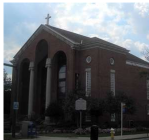
Alfred Street Baptist Church-Renovation
